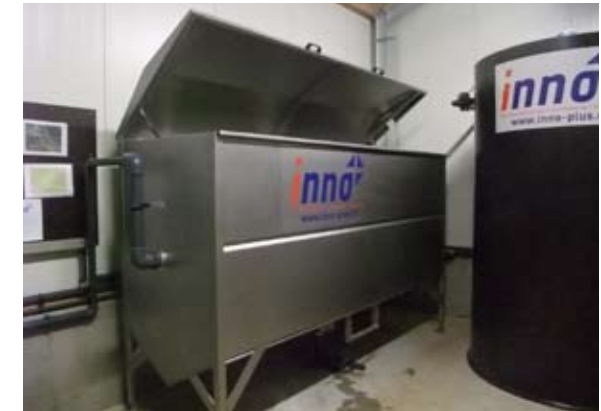
Inno+ Clean waterzuiveringsbak + denitrificatie reactor
